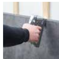
tiles: staple, nail, or glue
